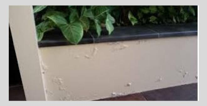
A common problem with walls and floors that are effectively underground or have earth back-fill against the external surface is that they range from being always damp to water seeping through them.
