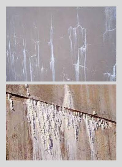
This can cause discolouration of paint or render burn, when moisture is coming from above it can even form Stalactites. Ensuring all horizontal surfaces have additional base coating system of a horizontal membrane such as Ardex WPM310 allows your substrate to be in is best possible preservation point, Tie these preparatory coats in with a product such as Dulux Acrashield which is also a membrane, you will have no problems ensuring a 10 warranty from supplies of products.
